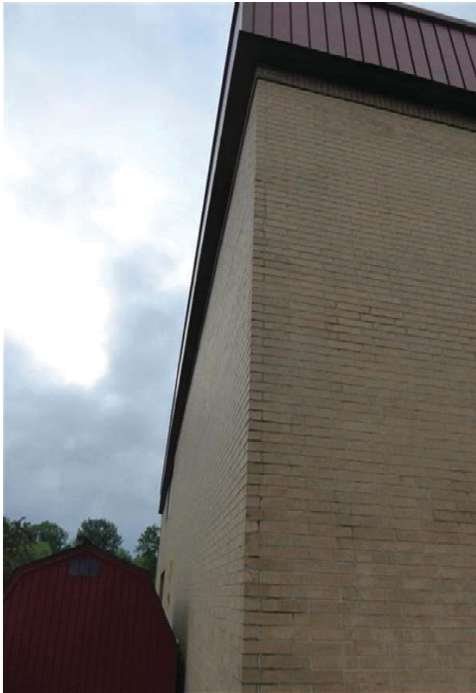
Photo 57 Vertical cracking was observed at several building corners creating a natural expansion joint.
