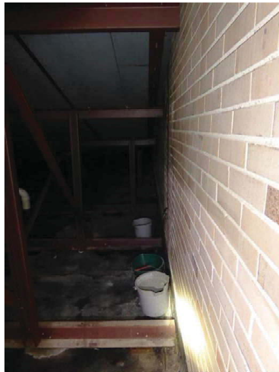
Photo 14 An active leak was observed in the attic near the northwest corner of the building.
