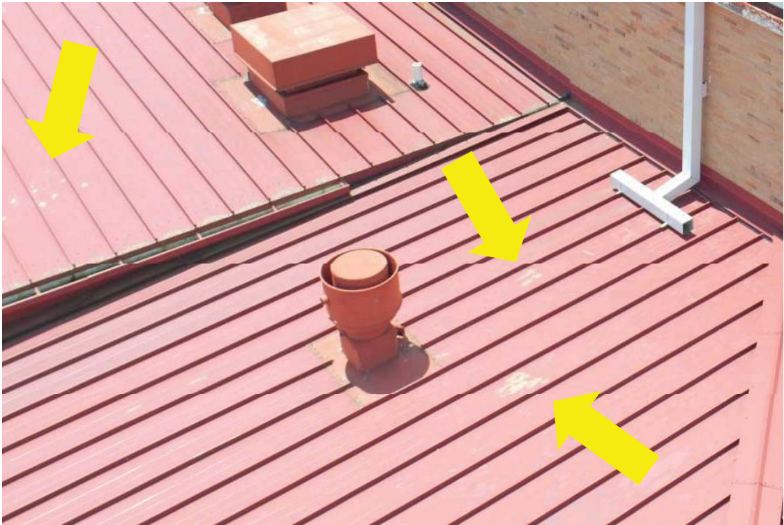
Photo 13 The red finish coat on the standing seam metal roof is worn in spots.
