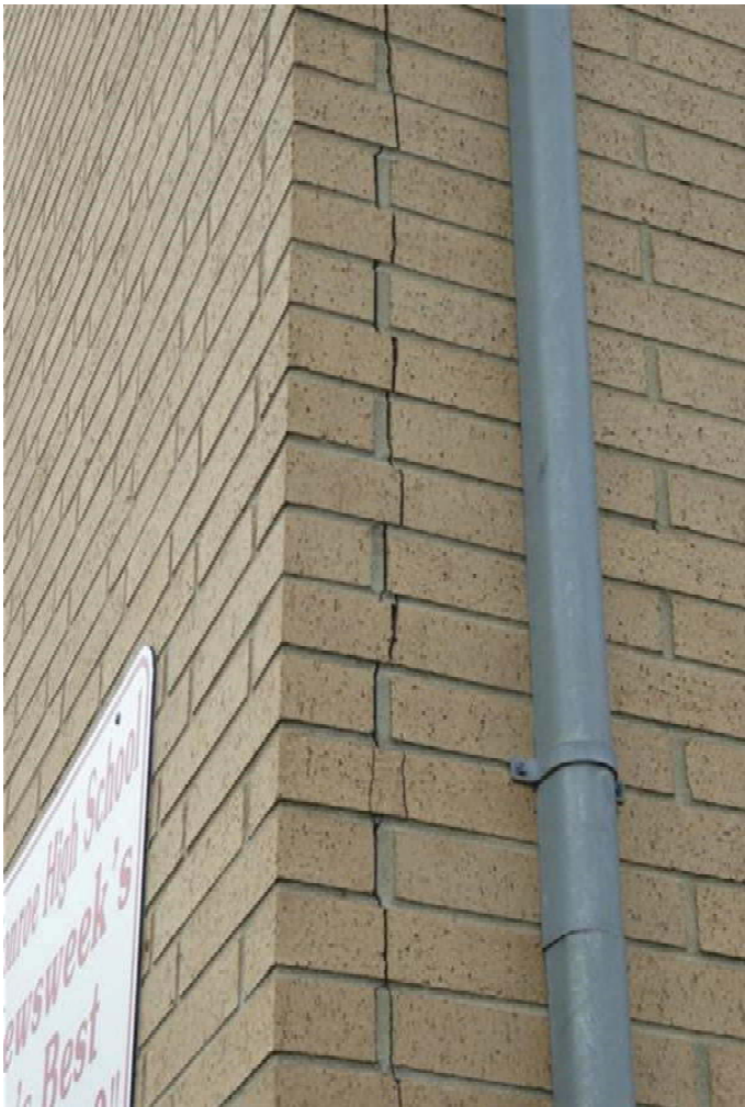
Photo 58 These should be saw cut and installed with backer rod and sealant to allow for expansion / contraction.
