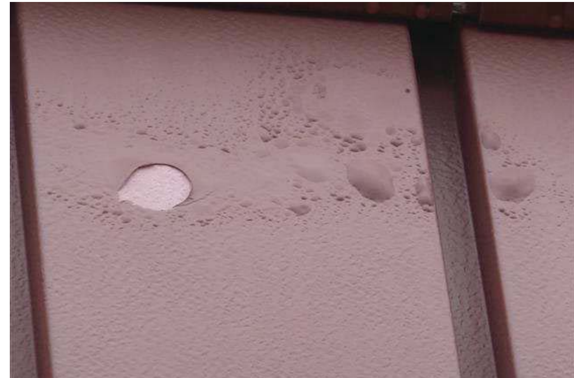
Photo 53 Paint blisters were also observed on metal fascia panels.
