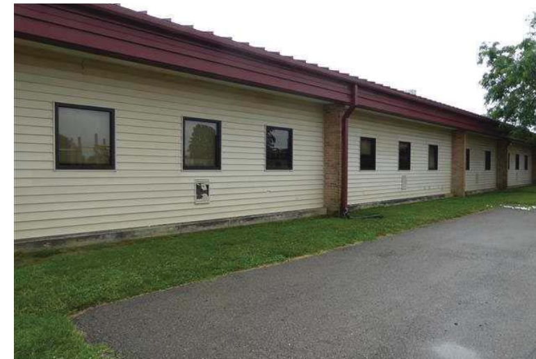
Photo 31 Vinyl siding clads much of the building.
